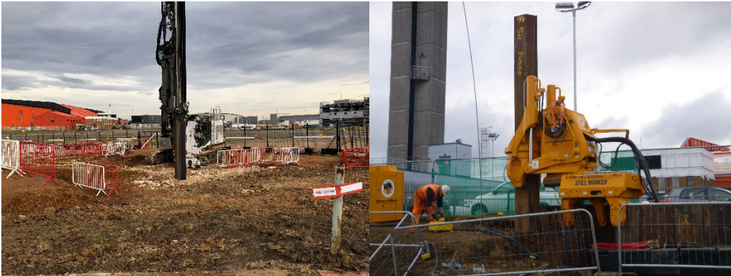
Inset 5.6: Typical sheet piling operation (right photo using silent piler)
